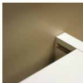
Base cabinets are 570mm deep with 49mm void. Internal depth 513mm
